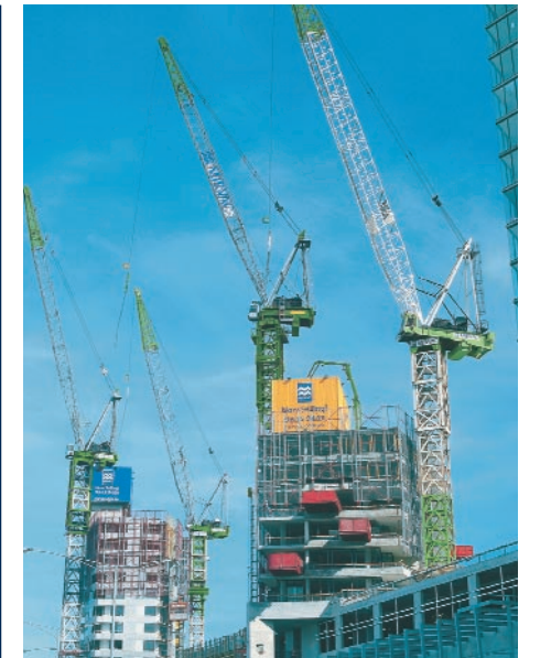
Melbourne's CBD and adjacent area has never seen such a demand for tower cranes, a large proportion are BOOM cranes.
