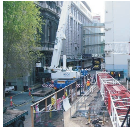
Assembling a 55 m. boom on an incredibly congested site - experience delivers a quick trouble free outcome.
